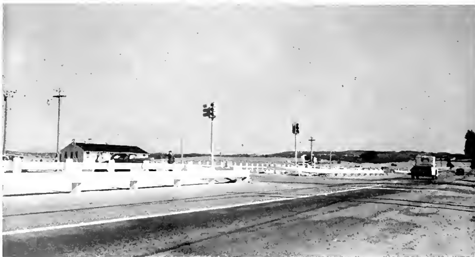
Turning movements restricted by use of metal guard rail at intersection where two roadways are at same level
